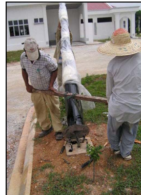
4. Place the pole onto the concrete stump
