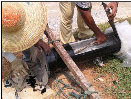
3. Insert the wire into the pole
