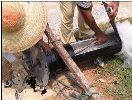
3. Insert the wire into the pole
