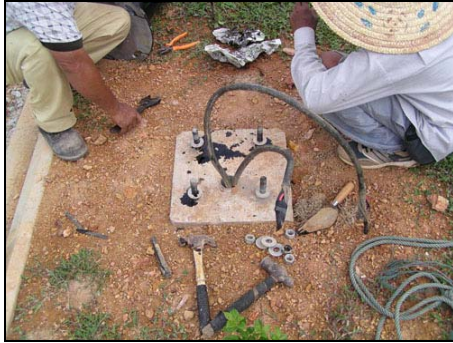
1. Prepare concrete stump c/w wire
